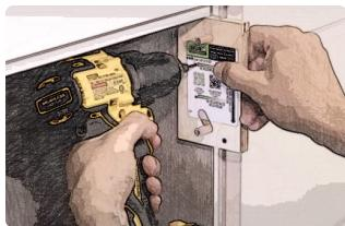
**F.** Secure top hinge plate first using screws labeled "Front Screws For Frameless Hinge Plates". Attach bottom plates to hinges on door.
