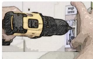
**C.** Secure top hinge first using screws from bag that says "Screw Hinges to Cabinet". When door is properly positioned, screw lower hinge into place. Apply rubber bumpers to corners of doors, opposite of hinges.
