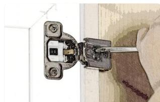
**D.** Adjust hinges to align doors making sure they close flush against cabinet. Adjustments move doors in and out and/or right and left. For up and down adjustment, loosen hinge on cabinet and slide hinge up or down.
