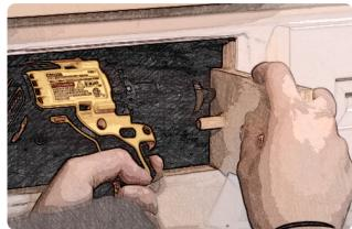
**B.** Use Phillips screwdriver to secure post using larger, #8x1" screw supplied, (manual screw driver is recommended for this step).
