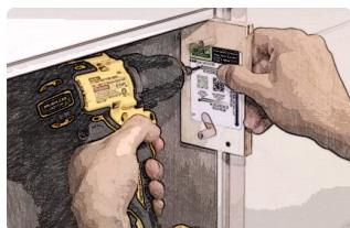
**F.** Secure top hinge plate first using screws labeled "Front Screws For Frameless Hinge Plates". Attach bottom plates to hinges on door.
