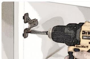
**G.** Clip top hinge to top hinge plate. When door is properly positioned, screw lower hinge plate into place. Apply rubber bumpers to corners of doors, opposite of hinges.
