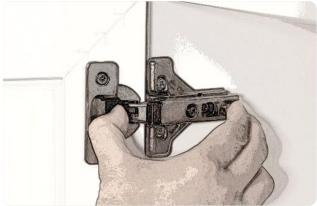
**H.** Adjust hinges to align doors making sure they close flush against cabinet. Adjustments move doors in and out and/or right and left. For up and down adjustment, loosen hinge on cabinet and slide hinge up or down.
